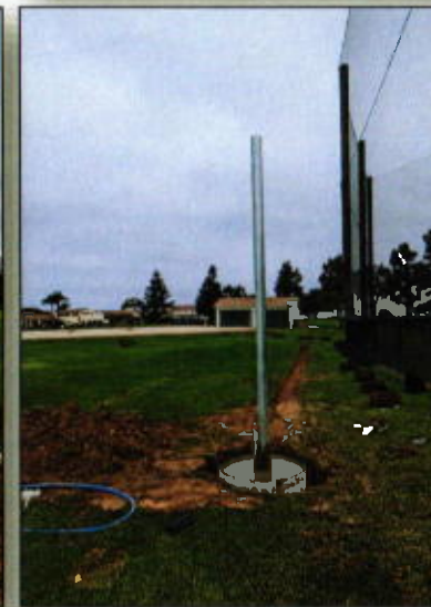
Concrete Poured Into 36" x 36" Sonotube
