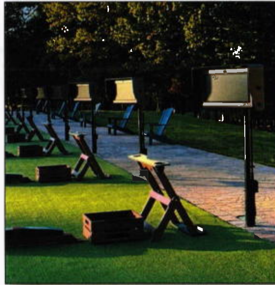
Examples of Individual Touchscreens at Hitting Bays with Power & Cat-6 Run Up the Pole
