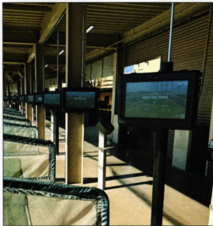
Examples of Conduit Run for Power and Cat-6 Bring Dropped to Each Screen from Ceiling
