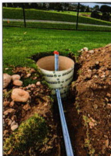
Conduit Stemmed Through Sonotube Cast
