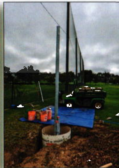
Pole Measured and Level Set along Conduit
