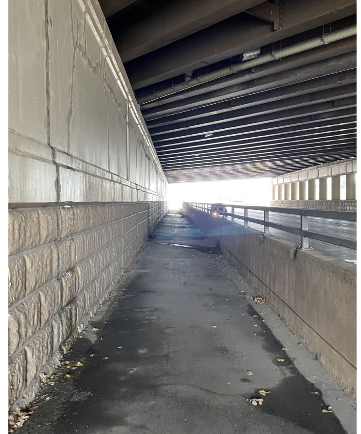
View underneath viaduct
