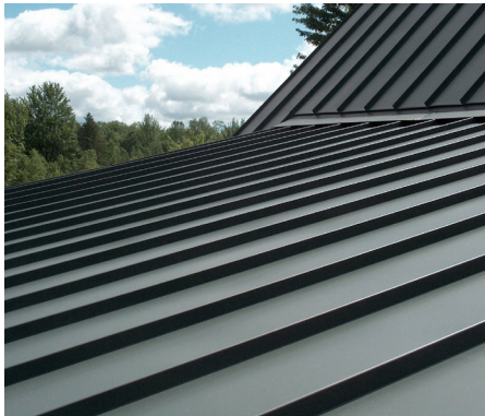
STANDING SEAM ROOF
