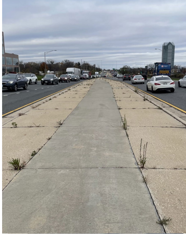
Concrete median on Kingery Highway
