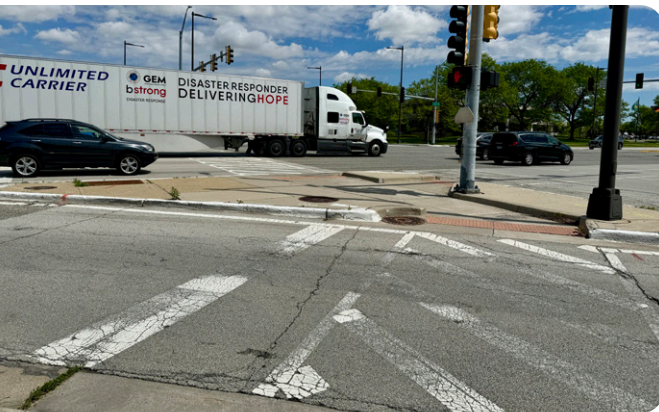
Intersection crossing at York Rd and 22nd St (southwest corner)
