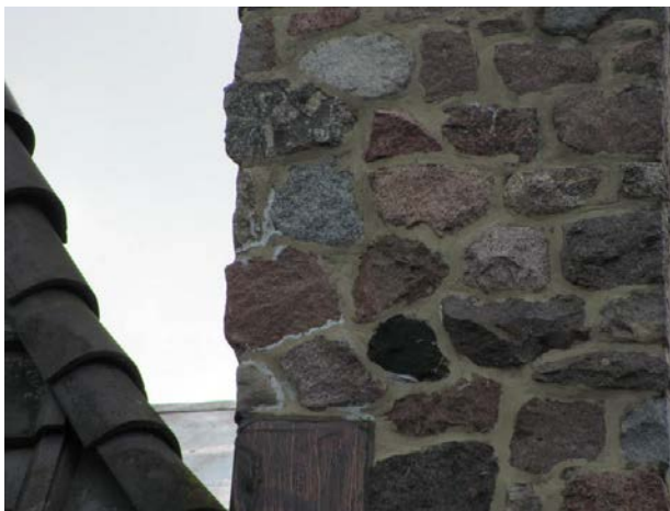
Efflorescence
