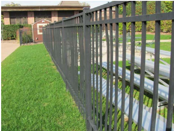
Aluminum pool fence, note bent pickets
