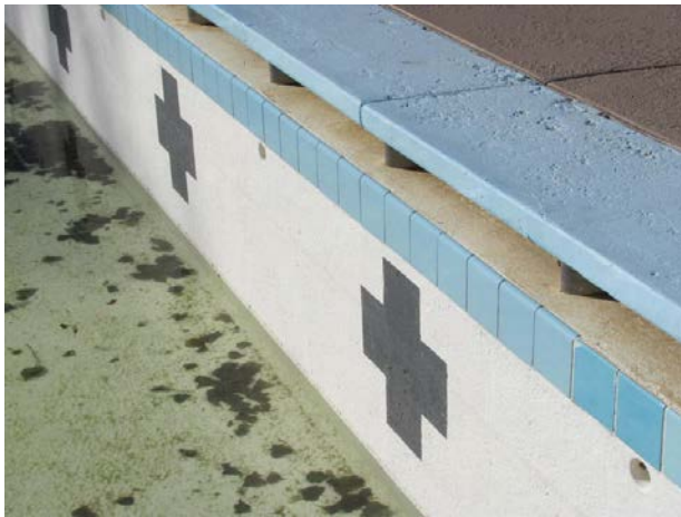
Paint finish at lap pool
