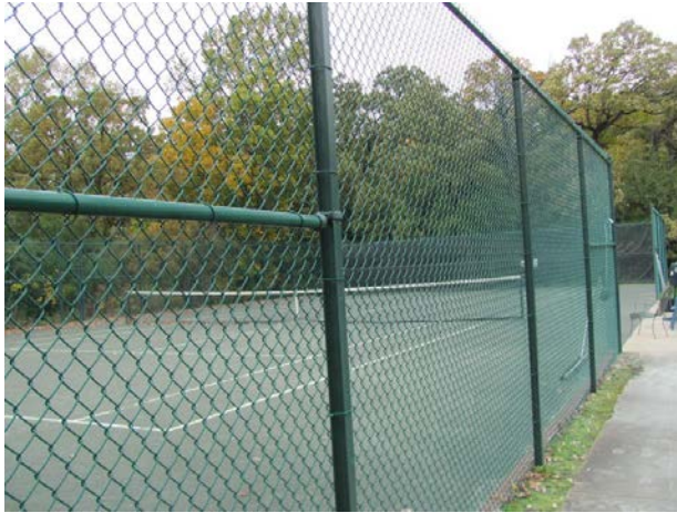
Newer chain link with painted older posts at courts 1 and 2
