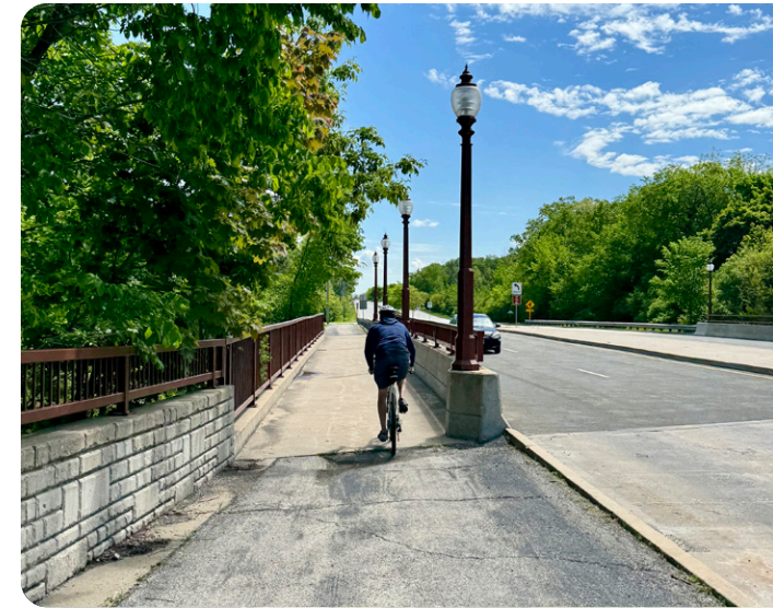
Path and bridge along 31st St at Salt Creek
