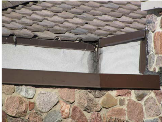
Modified bitumen roof
