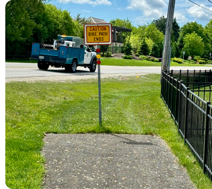
End of sidepath on York Rd
