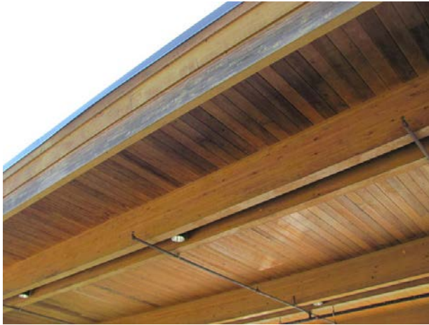
Wood soffit at porte-cochere
