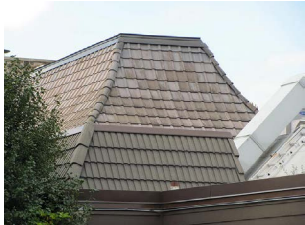
Older and newer concrete tile roofs
