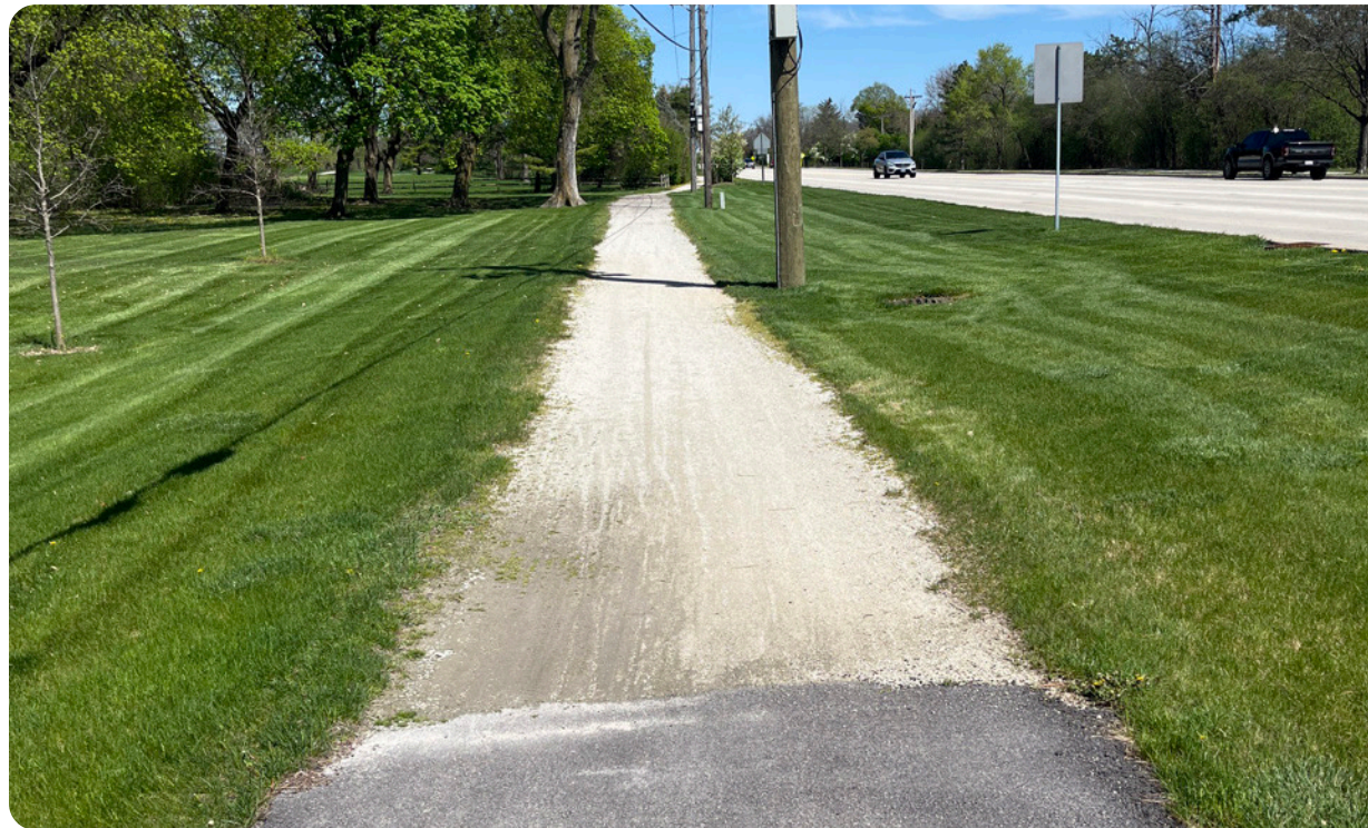
Existing path along York Rd near Butler National Golf Club
