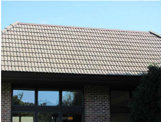
Concrete tile roof at addition
