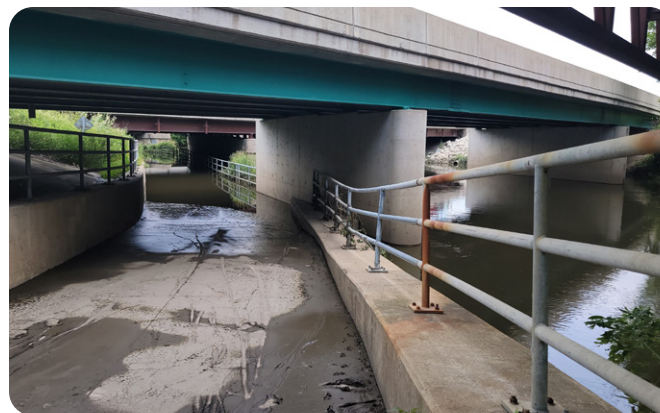
Salt Creek Trail underpass beneath Roosevelt Rd
