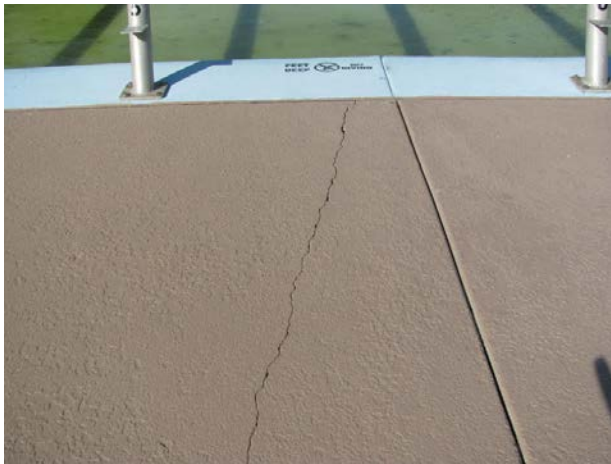
Concrete crack
