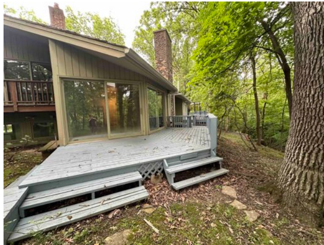
VIEW LOOKING SOUTH OF EXISTING WOOD DECK
