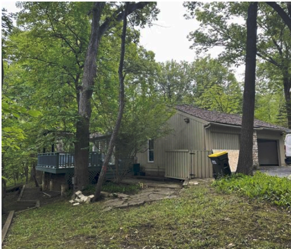
VIEW LOOKING NORTH OF EXISTING WOOD DECK
