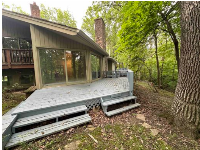
VIEW LOOKING SOUTH OF EXISTING WOOD DECK
