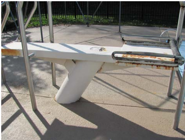
Typical rust at diving stand
