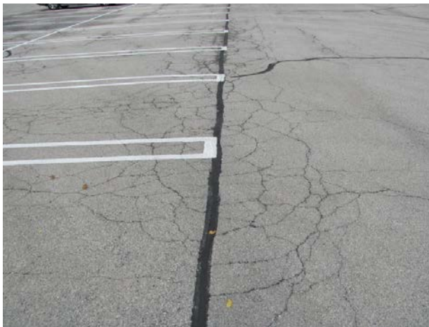
Alligator cracks
