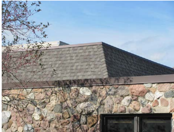
Asphalt shingle roof
