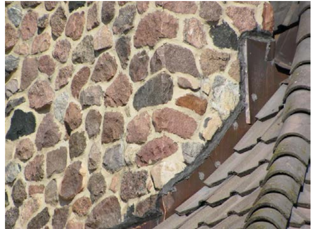
Sealant and flashing at chimney and roof
