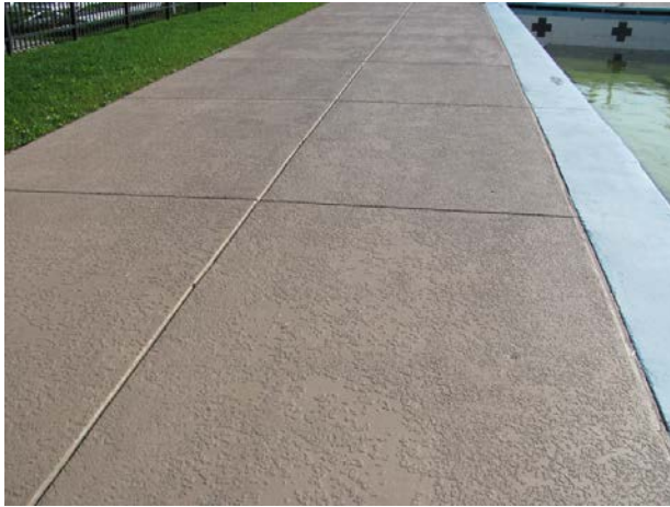
Coated concrete deck
