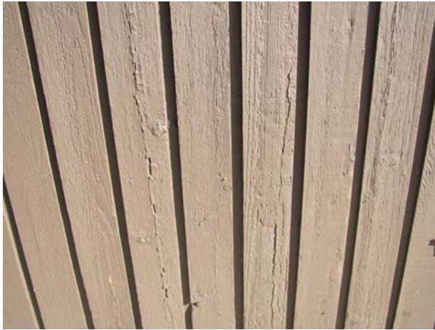
Typical weathered wood at original building
