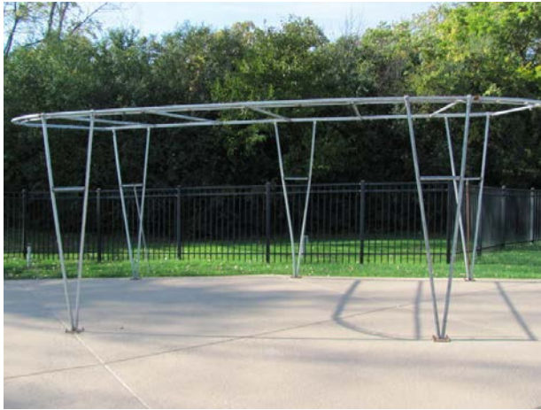
Shade structure metal frame
