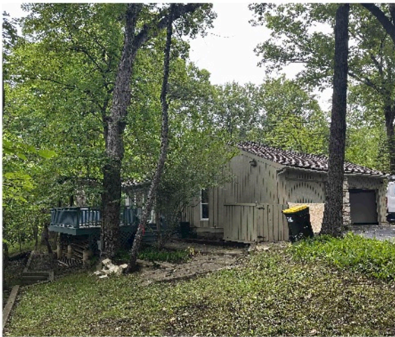
VIEW LOOKING NORTH OF EXISTING WOOD DECK
