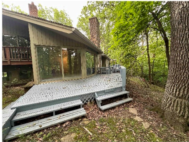
VIEW LOOKING SOUTH OF EXISTING WOOD DECK
