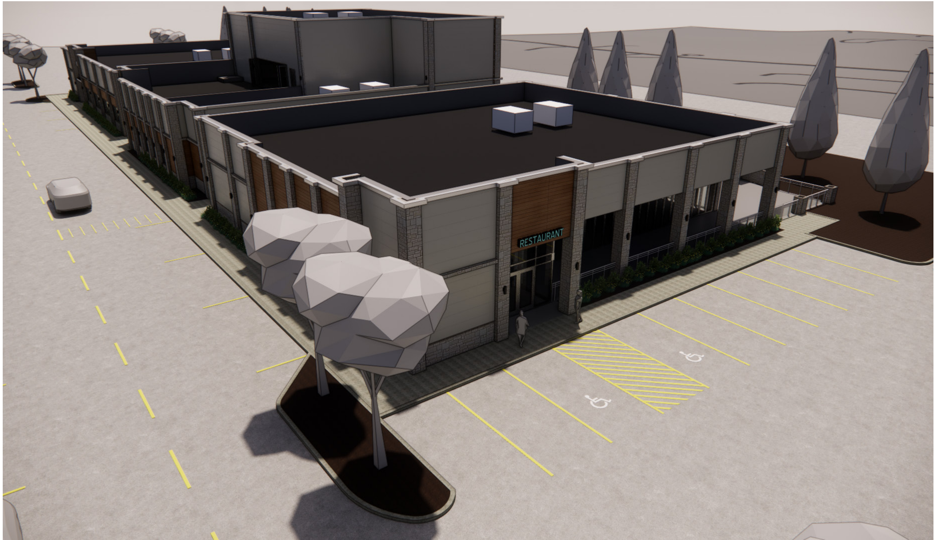
Elevated view - Looking Southeast from Northwest corner of Pad G
