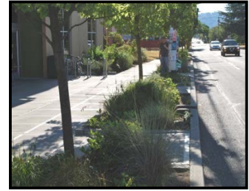
Stormwater runoff is treated in a series of rain gardens within the parkway of this urban street section
