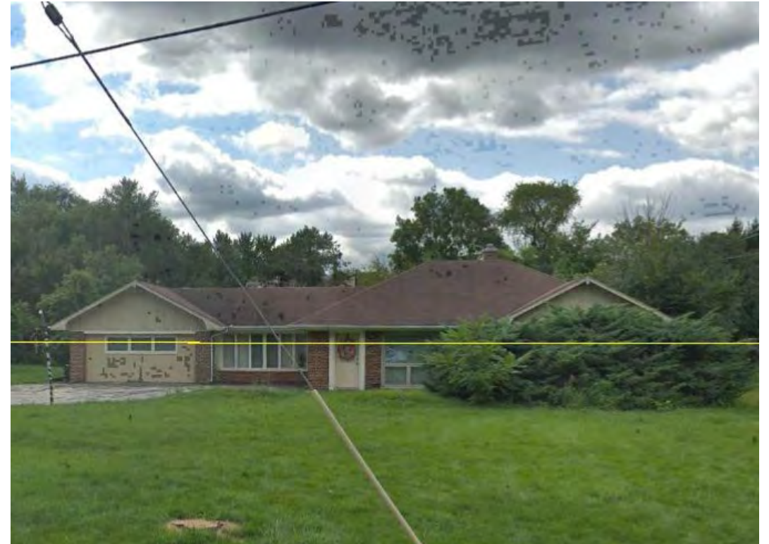
NORTH NEIGHBOR TO BE DEMOLISHED
